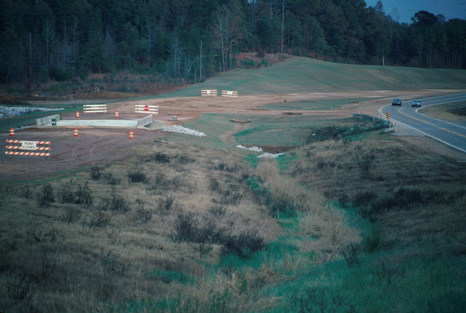
Highway construction with visible BMPs: mulching, seeding, rock check dams.
